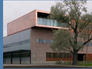
Aurora 2, Joensuu university building 8,100 m 2 2006 202 kWh/(m 2 a) 1) The building is U-shaped. There are glazed courtyards for the distribution of daylight to the surrounding office spaces in both wings.
