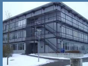
Multi Purpose Building, Stuttgart university building 9,150 m 2 1995 256 3) kWh/m 2 The building is used to help research groups overcome shortages of both office or laboratory space. Energy performance in the multi-purpose building is quite poor due to the laboratories.
