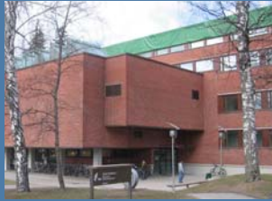
Engineering department, Espoo university building 8,600 m 2 1966 275 kWh/(m 2 a) 1) The building comprises offices for researchers, auditoriums, seminar rooms, classrooms and a canteen.
